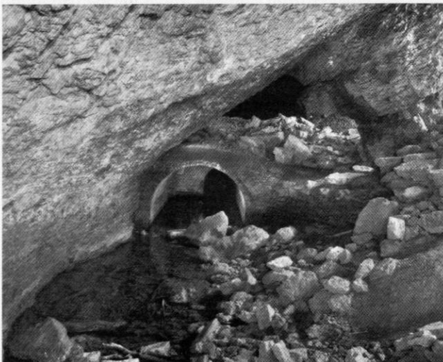
The lower gallery of Dark Cavern, Castle Hill in 1986, looking north in the thick bed limestone. The canal runs along the footwall of the mine. The Dark Cavern has now been filled with sand. Photo by Nick Catford
